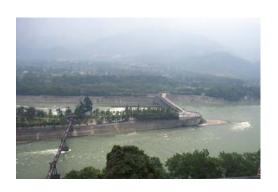
**D**ujiangyan is an irrigation infrastructure built in 256 BC during the Warring States Period of China by the Kingdom of Qin. It is located in the Min River near Chengdu. It is still in use today to irrigate over 5,300 square kilometers of land. The Dujiangyan along with the Zhengguo Canal in Shaanxi Province and the Lingqu
